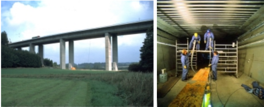
Fig. 2: Valley bridge Kronsdorf
