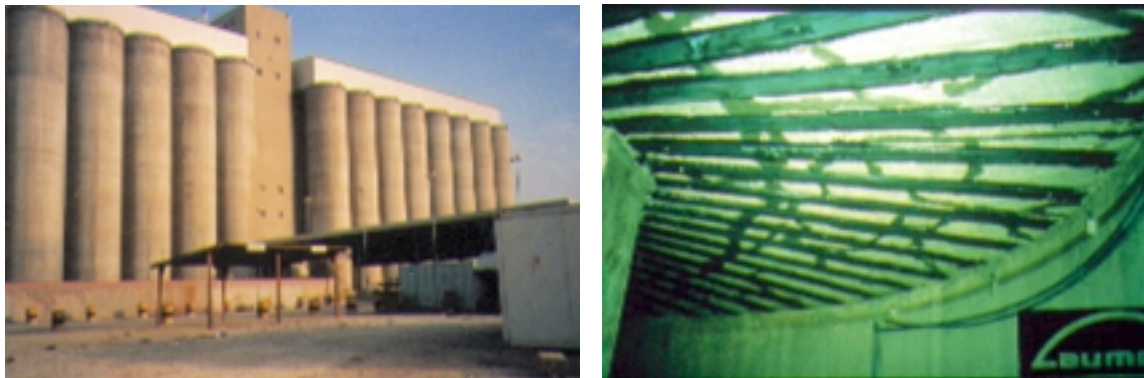
Fig. 1: Large silo works near Rhyad
